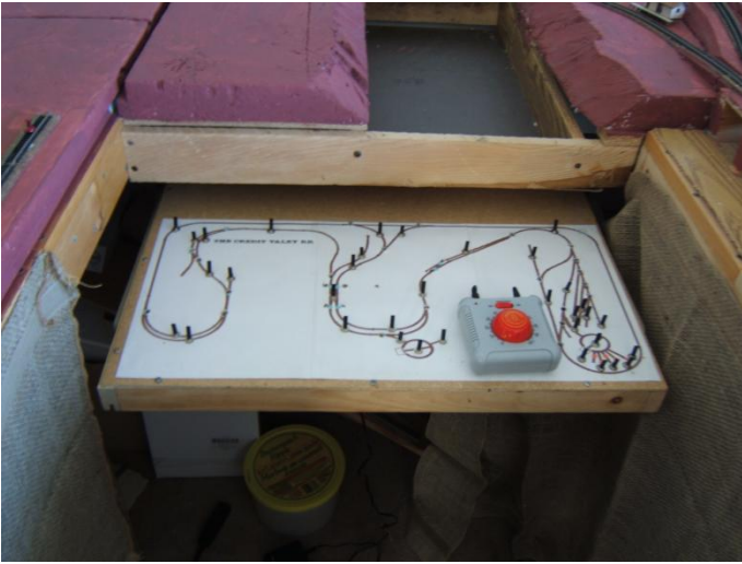
Original Main CVR Control panel, Forks of The Credit station can be seen in the upper right corner
